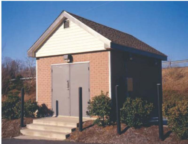
Generator building, Oliver City Sanitary Sewer System Warrenton, VA
